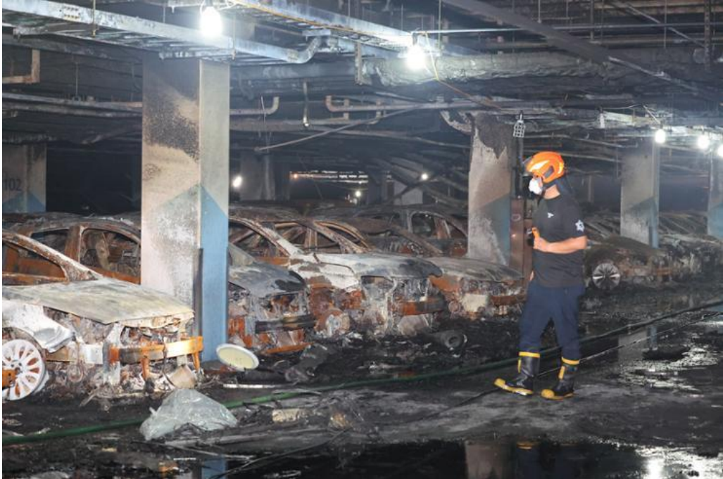
Apartment Car Park, South Korea, 2024
